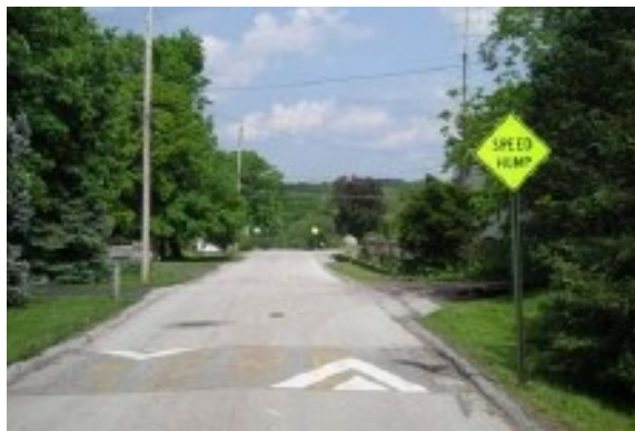
Strategically placed speed humps can be an effective traffic calming measures on rural roads.
