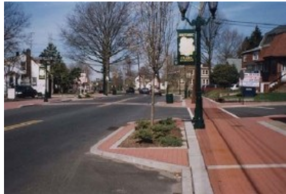
Vegetated curb extensions can shadow on-street parking and increase pedestrian visibility at busy intersections.
